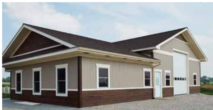
Featured: LP SmartSide Panel, Cedar Texture Shakes (staggered), Trim and Fascia
